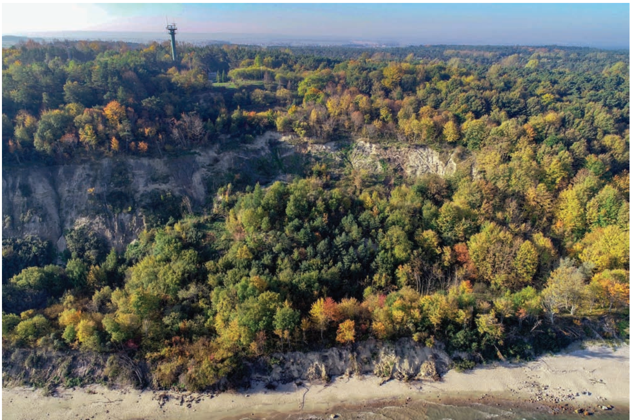
Fig. 4 Chłapowo cliff section and the landslide (photo: M. Olkowicz)
