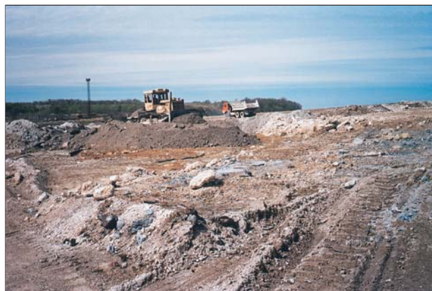
Fig. 4. Protection works in Sillamäe tailings pile in May 2003. Photo by A. Raukas.
