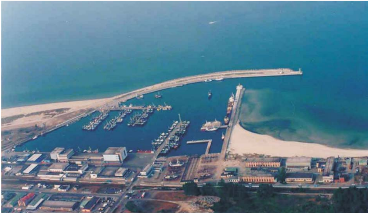
Fig. 2. General view of Władysławowo harbour (photo by J. Kapiński, 2003).
